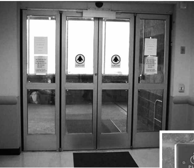
Automatic opening doors allow students using mobility devices to enter and exit without help as well as satisfying security concerns.
